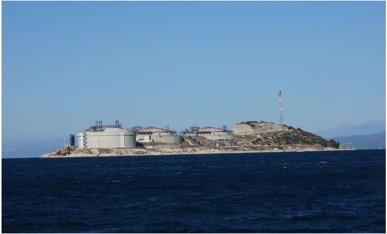
Fig. 2. Revythousa Island is nearly completely occupied by natural gas storage facilities and was not surveyed
