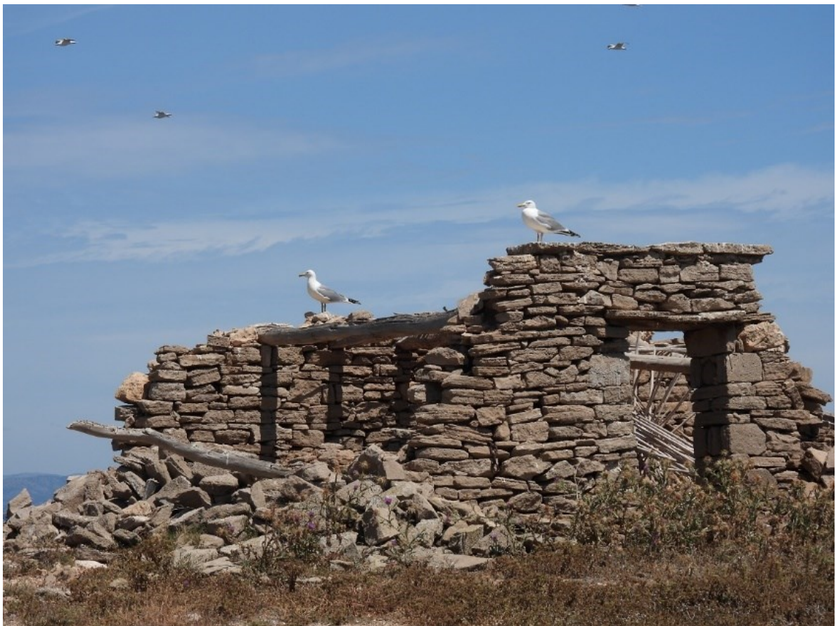
Fig. 21. Abandoned old buildings on Metopi Islet
