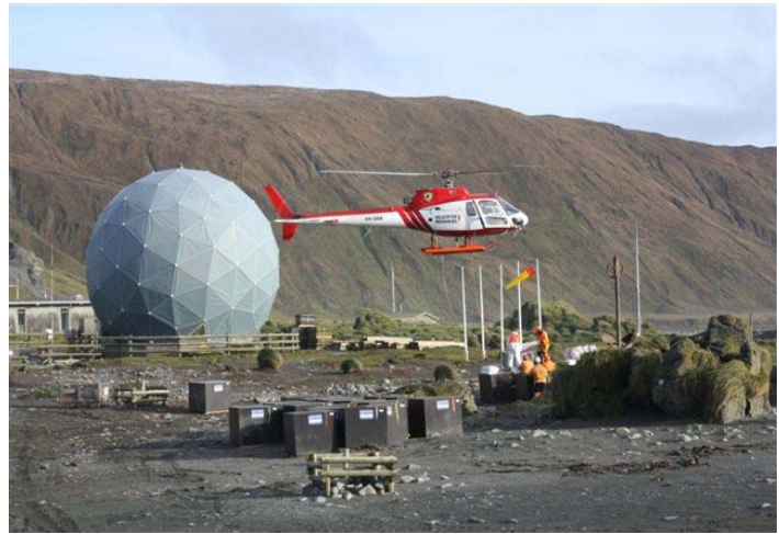
Dome housing the communications satellite dish.
