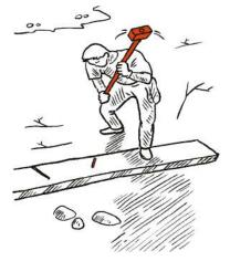
**STEP 4:** Fix the step to the ground by hammering in the reinforcement bars (10 cm on hard substrate; 40 cm on soft substrate and up to 1 m in sand).
