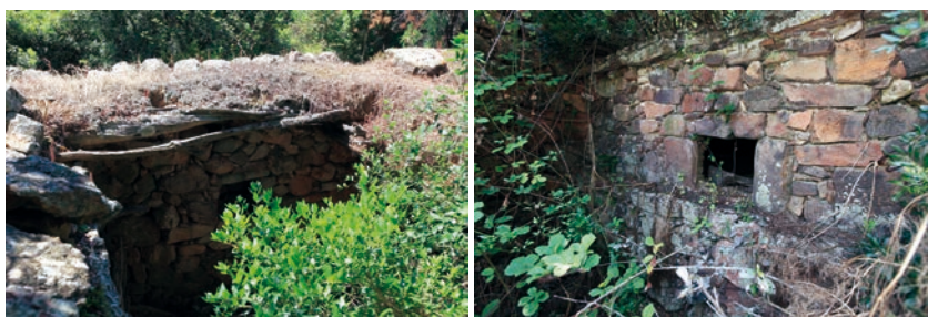
Figure 7. Left. A cellar under shelter ( 'u palmentu' ) for the fermentation of grape juice into wine at L'Elbu. Note the roof covered with earth. Right. A bread oven ( 'u furnu' ), in the wall of a stone hut. Photos © Jean-Marie Dominici.
