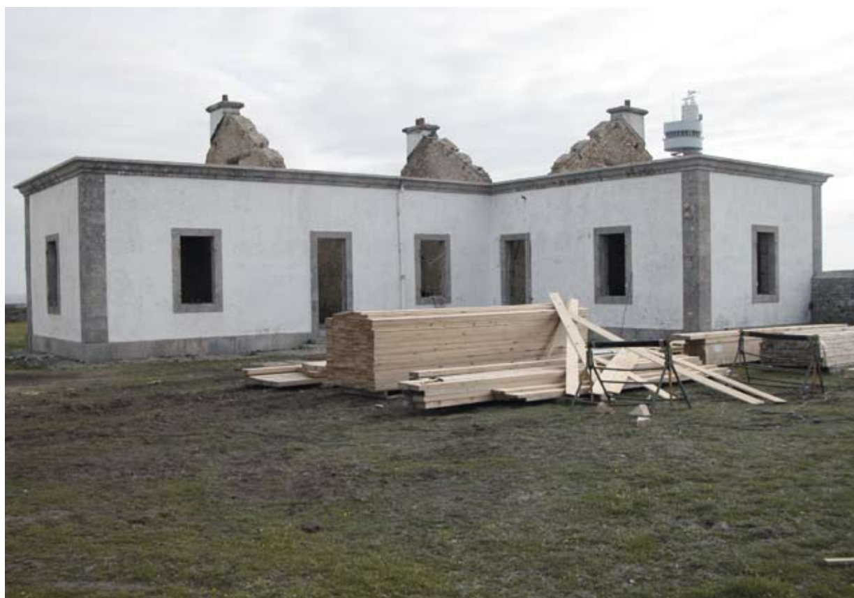
Quisant, Stiff house rebuilding
