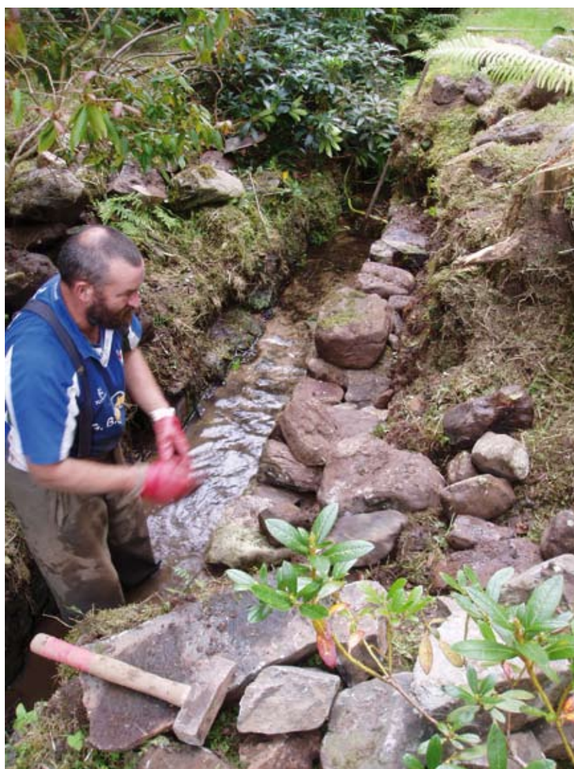
Argyll & Bute, Ha-Ha wall restoration
