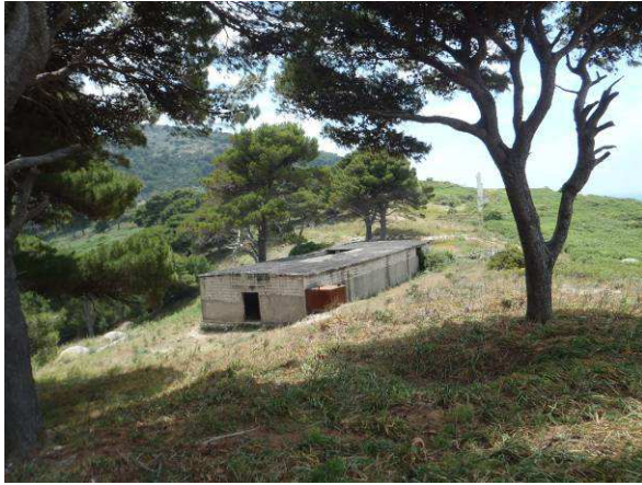
Location 21: Ground floor impair masonry construction. Metal : 0.3 ton
